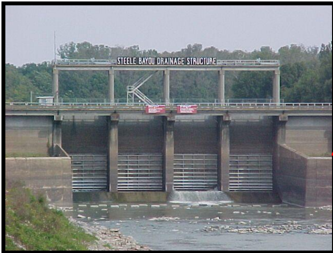
Steele Bayou Drainage Structure
