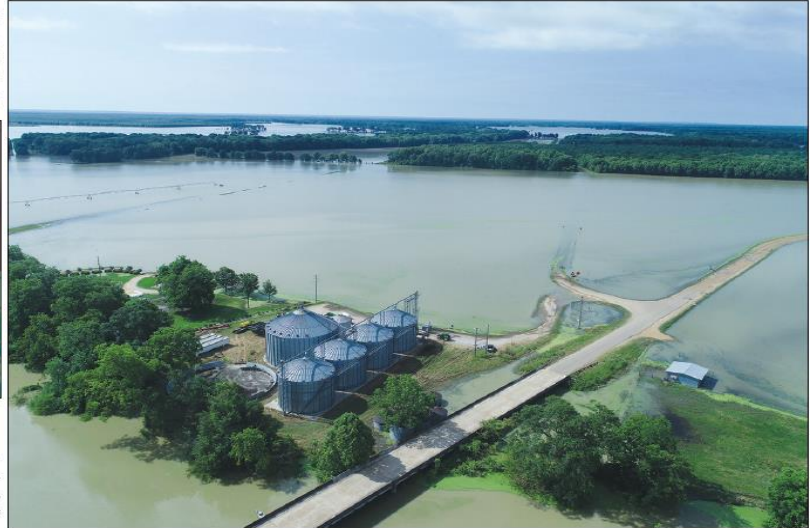
Aerial drone images of Holly Bluff Road at the Big Sunflower bridge from May 30 shows just a small part of the more than 500,000 acres still inundated with floodwaters mid-June. With less than predicted rainfall and an equalization of the water on both sides of the Steele Bayou Draining Structure, the U.S. Army Corps of Engineers announced Wednesday morning that the structure's gates would be opened sometime during the day.
